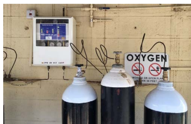
A cylinder-based manifold system in Kenya. Photo: PATH/Lisa Smith.
