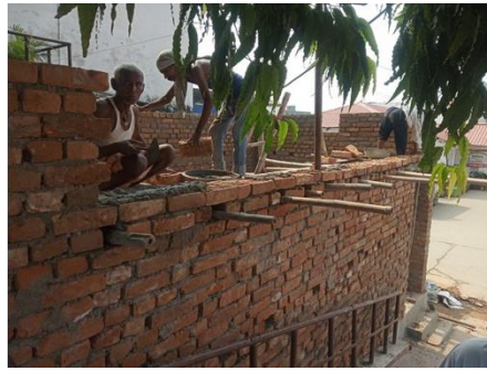
Figure 2: Construction of a central manifold room at Sadar Hospital
