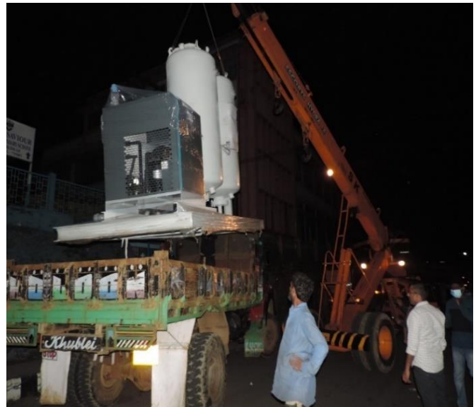
PSA plant being installed in Nazareth Hospital
