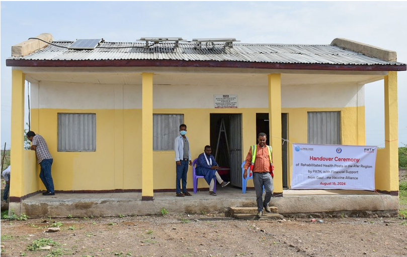
A renovated health post during its August 2024 handover ceremony. PATH and Gavi, the Vaccine Alliance supported repairs to help restore health services in conflict-affected areas.
