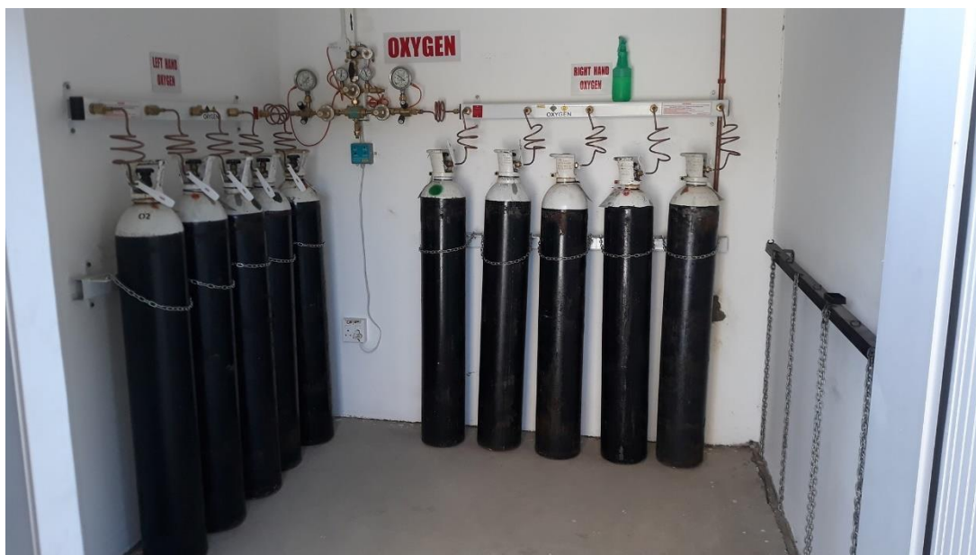
Fig 2: Manifold system
