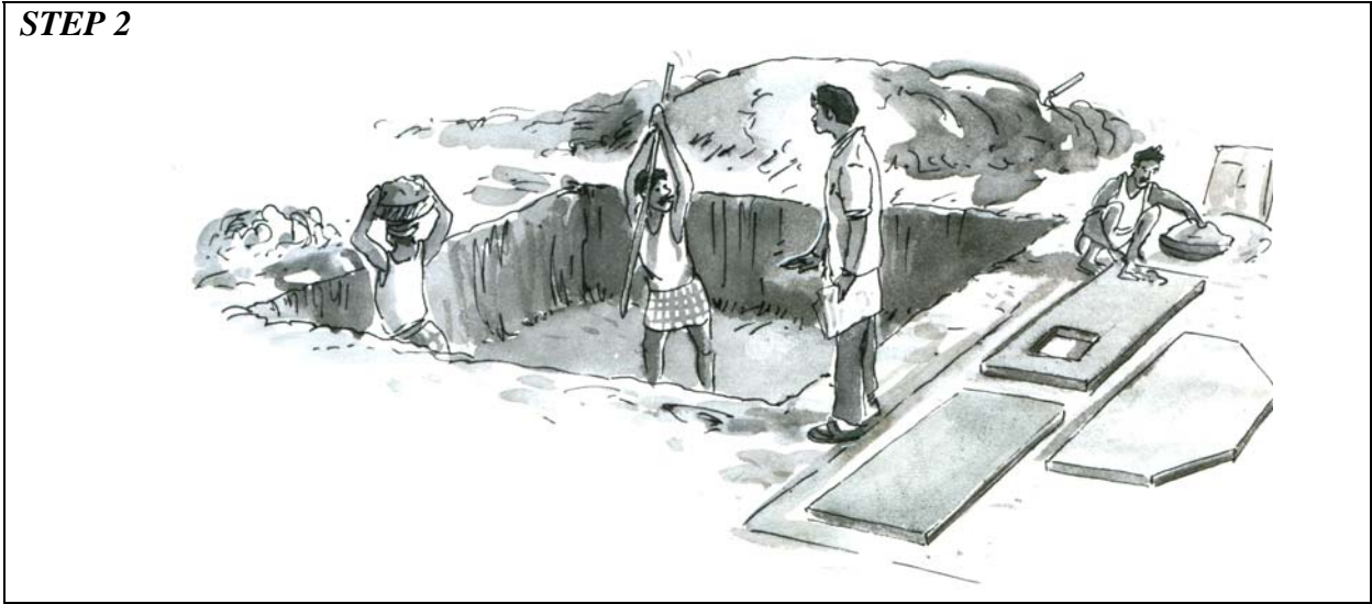
Figure 2.3.2 Digging WDU foundation and ash pit
