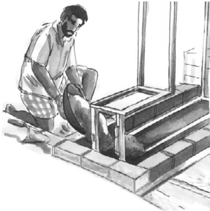
Figure 2.3.5 Placing metallic frame and grouting frame in PCC slab
