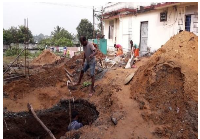
Site work is in progress for civil work in Bijapur, Chattisgarh
